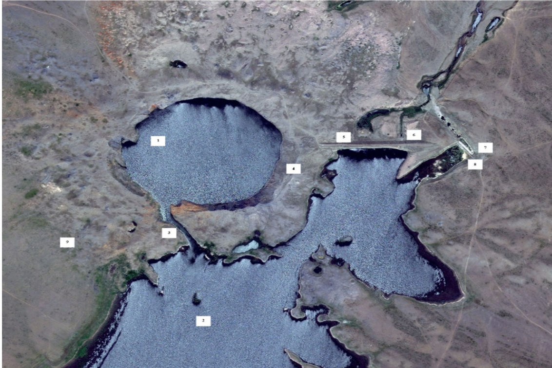
Figure 1. Scheme of artificial water reservoir on Shagan river and assembly of its structure. 1 – Internal reservoir; 2 – External reservoir; 3 – Water supply canal; 4 – Dump of ground; 5 – Rock-fill dam; 6 – Bottom drain; 7 – Flow side spillway with side weir; 8 – The remains of destroyed dam; 9 – Border of dump of soil [1].
